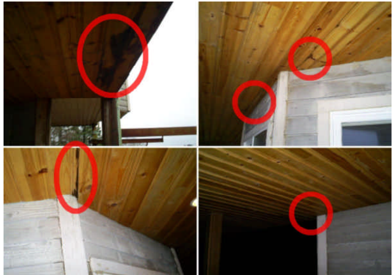
Deck soffit moisture stains
