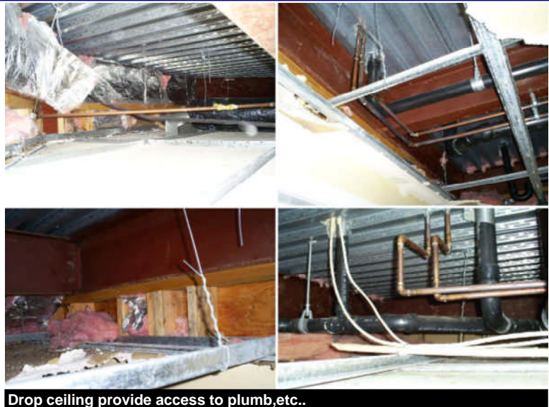
Drop ceiling provide access to plumb,etc..
