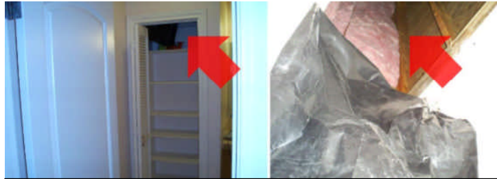
Attic Access. No Hatch cover.
