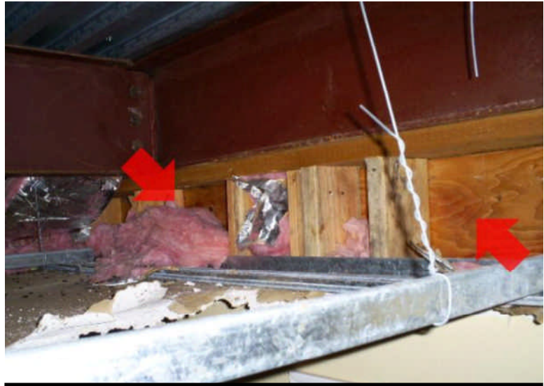
Exterior wall insulation removed/fallen
