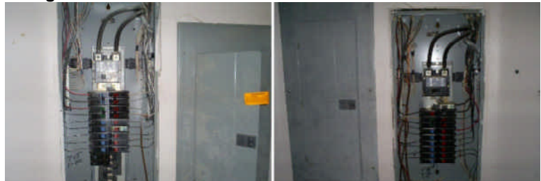
Both Panels wired as "Mains"
