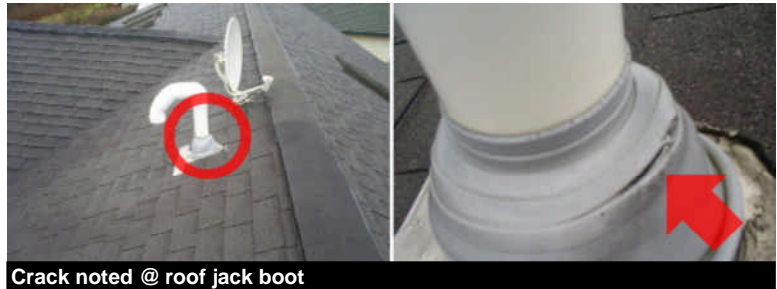
Crack noted @ roof jack boot
