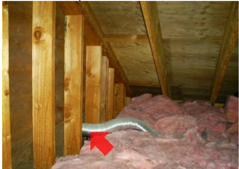
Bath exhausts to exterior=good
