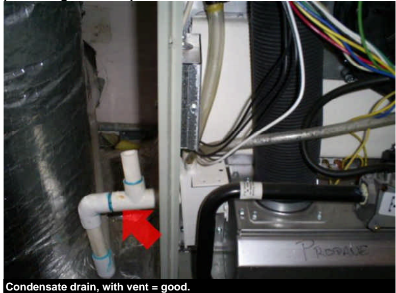
Condensate drain, with vent = good.
