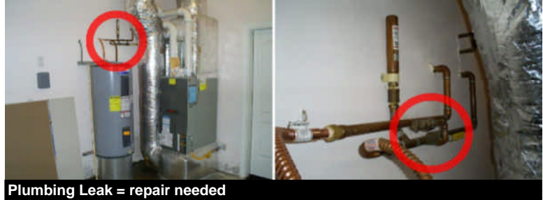
Plumbing Leak = repair needed
