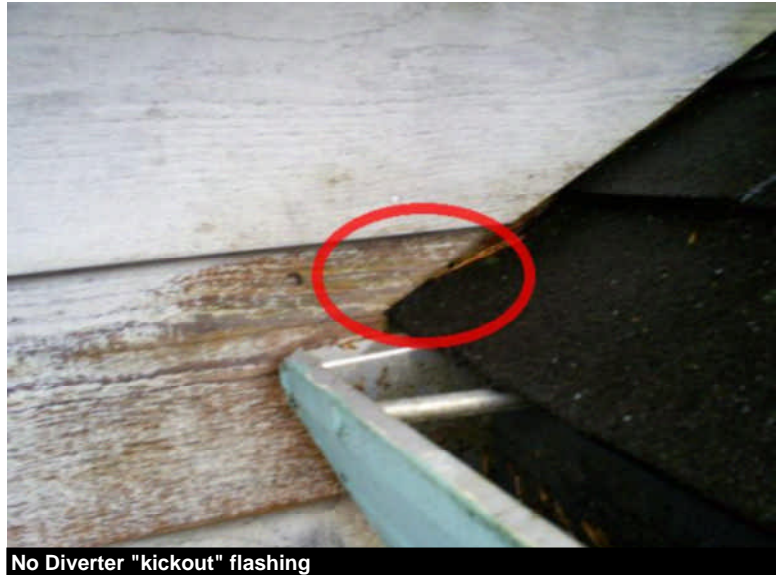
No Diverter "kickout" flashing
