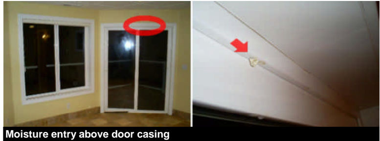
Moisture entry above door casing
