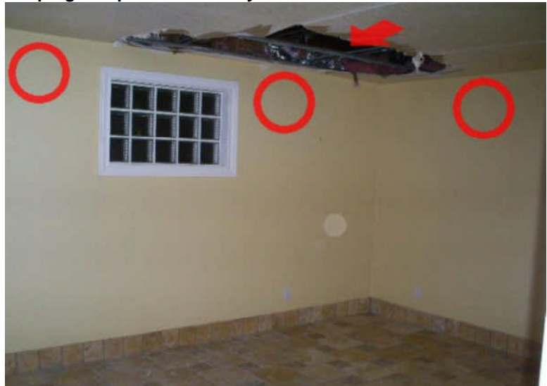
Paint sag=moisture. Ceiling Damaged
