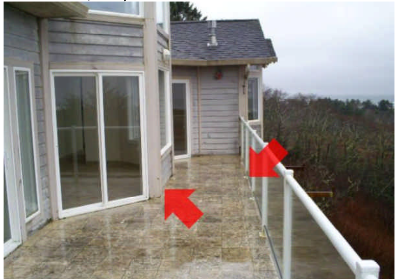
House joint, edge flashings inadequate
