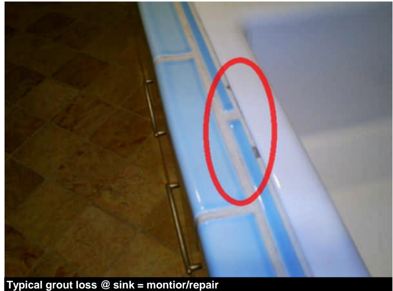
Typical grout loss @ sink = monitor/repair
