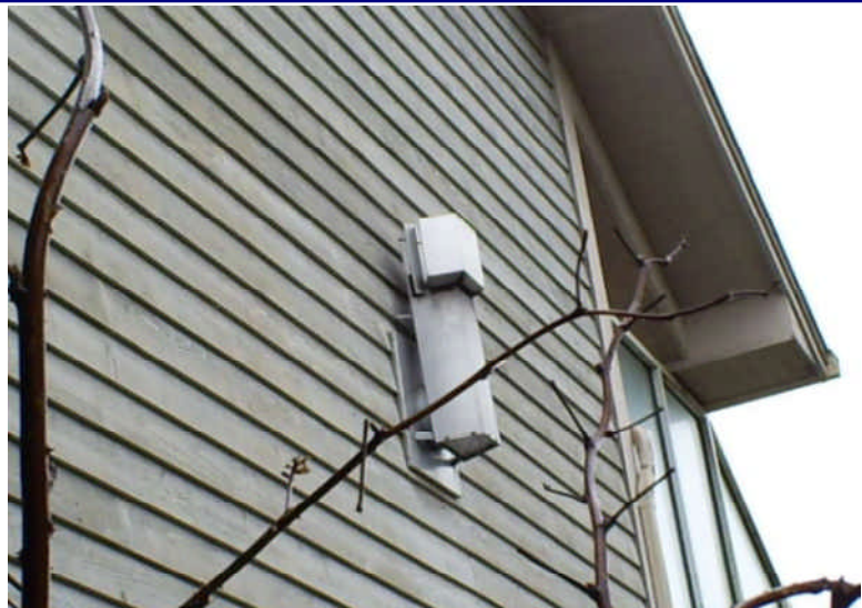
Direct vent flue for Gas Fireplace
