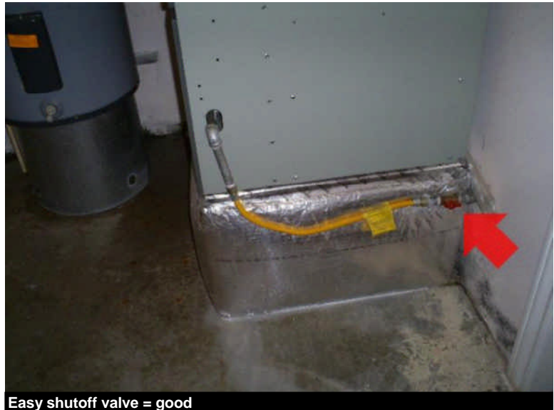
Easy shutoff valve = good
