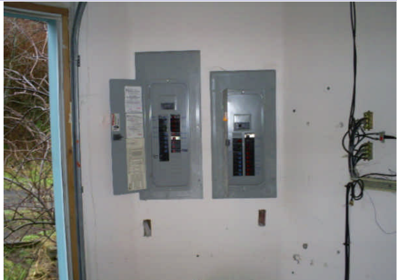
Panels wired as "Main" panels Garage.
