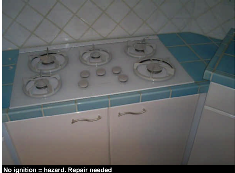
No ignition = hazard. Repair needed
