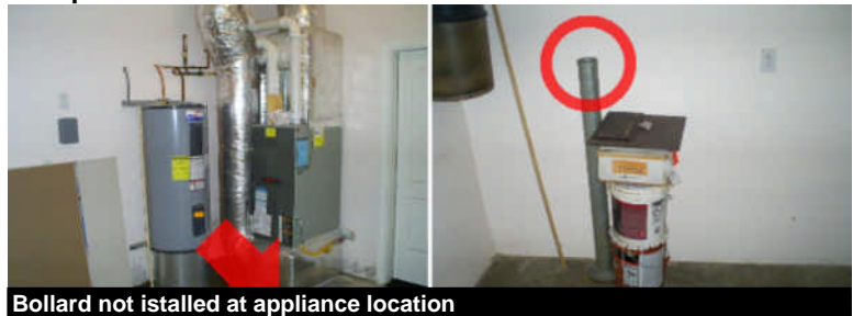
Bollard not installed at appliance location
