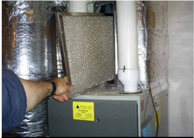
Filter located above unit
