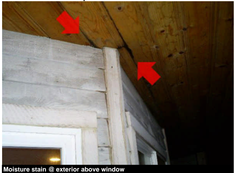
Moisture stain @ exterior above window
